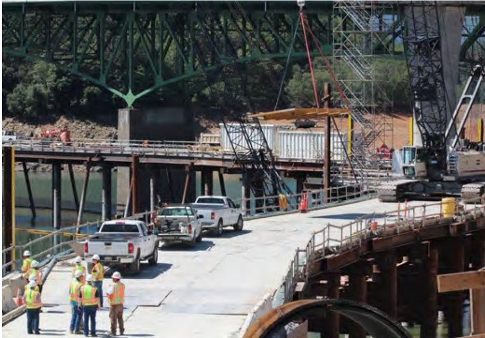
Figure 8 Antlers Bridge construction
